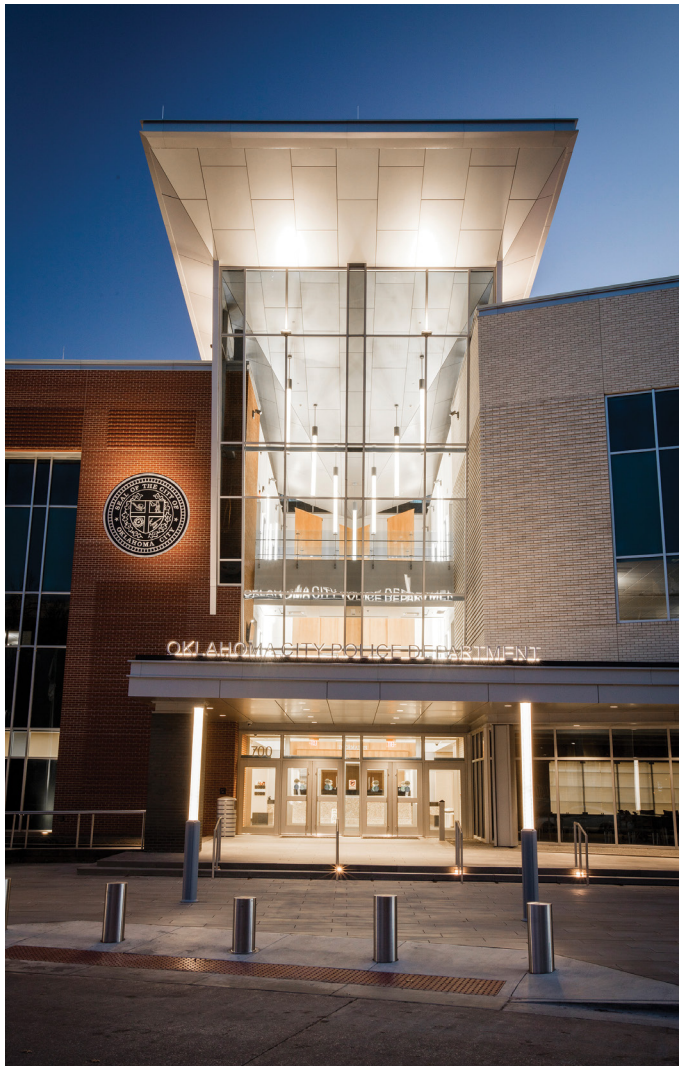
Sitting atop the 88,625-square-foot headquarters is a sloped diamond-shaped metal atrium roof—or “hat”—that is an iconic identifier for the downtown area.
