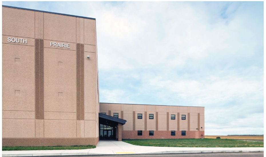
Precast concrete panels were used for a majority of the building shell to maintain a cohesive appearance between the existing school and the new addition.
