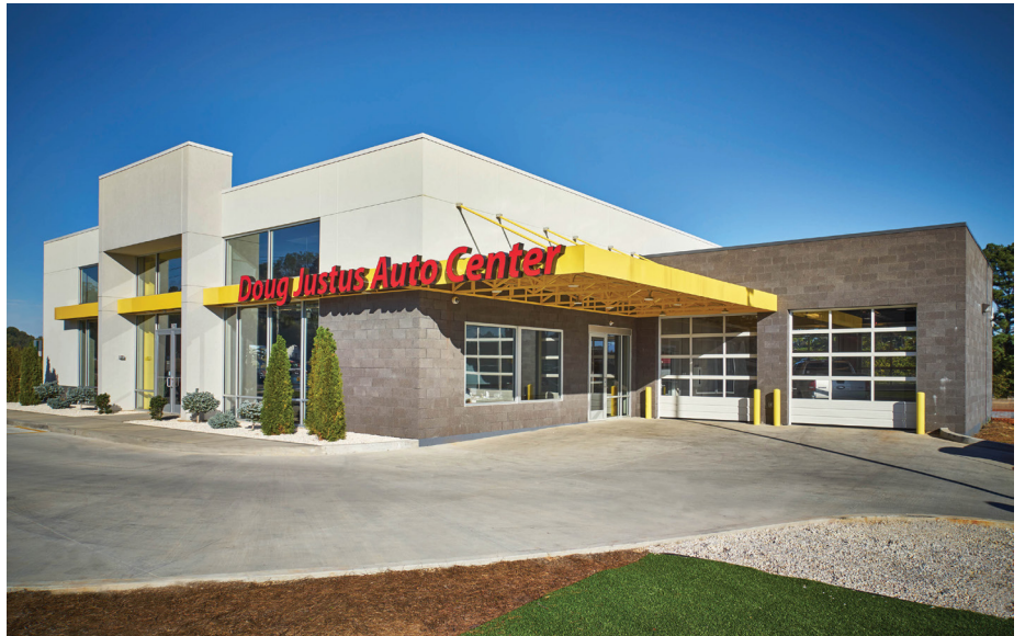
The illuminated red letters against the bright yellow custom canopy at the front of the building fit the sleek design of the space, and reflect the Doug Justus brand.
