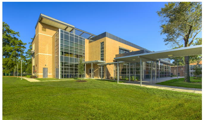
By linking the project to adjacent buildings via covered walkways, service access to all buildings was improved.
