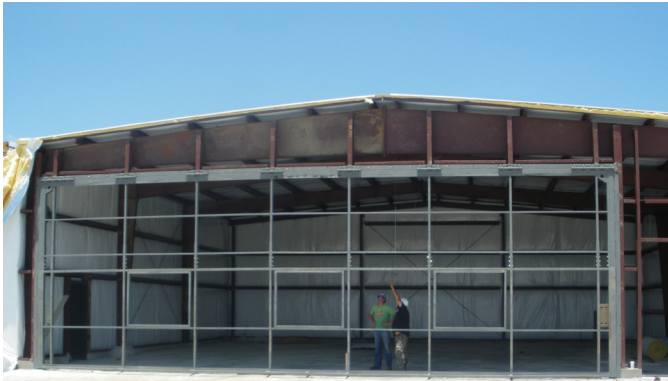
Architectural requirements for uniformity only allow hydraulic doors on Aero Country East hangars.
