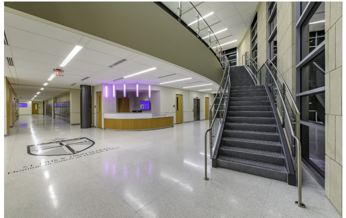
A distinctive composition of angled projections highlights the shared social spaces and stairways on the north and south elevations.
