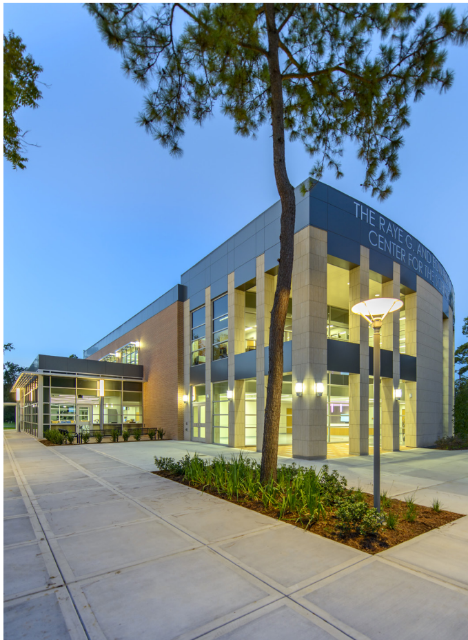
The new two-story complex provides a unique state-of-the-art learning environment for teaching the sciences.
