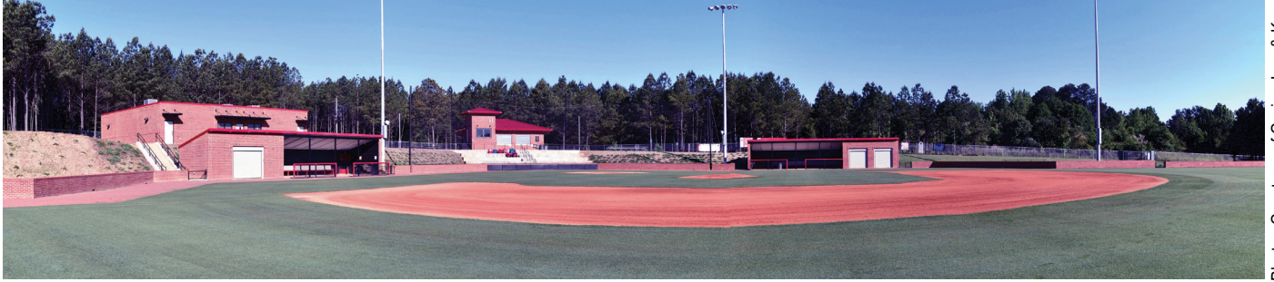
The baseball field, dugouts, concession building, fieldhouse, and hitting facility are all components of the baseball complex.
